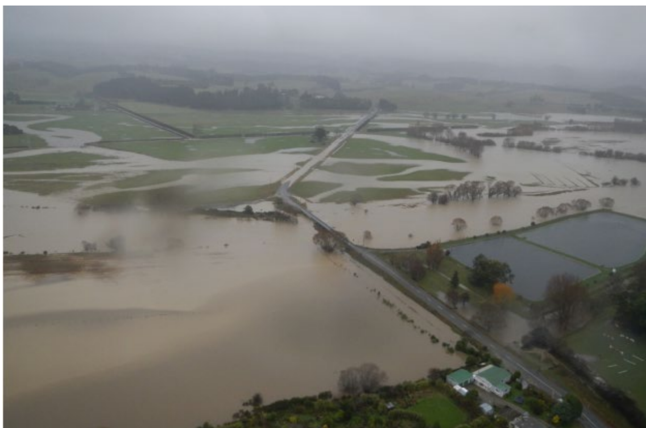
Figure 5: Waihemo/Shag River in flood, looking downstream at Horse Range Road bridge and Palmerston Wastewater Treatment Plant, 17 June 2013. Source: Williams et al. (2018), ORC.
